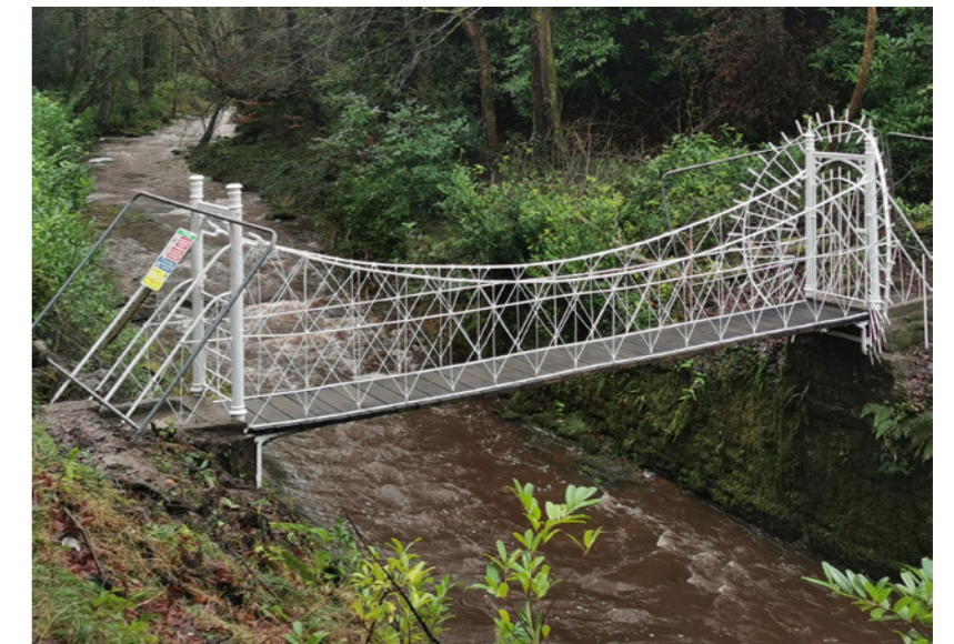
Kinnitty Suspension Bridge, conserved 2021. Photograph: Rachel McKenna
