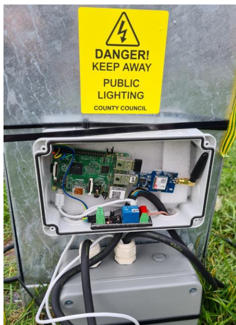
Figure 10: Relay installed at 'pop-up' section of lighting - Claddagh Basin Galway
