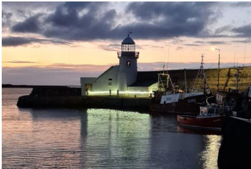
Figure 1: Trial installation at Balbriggan Lighthouse, Fingal - May 2022
