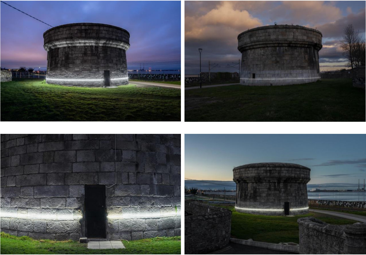
Figure 18: Martello Tower, Dún Laoghaire Rathdown (source: Pekka Niittyvirta)
