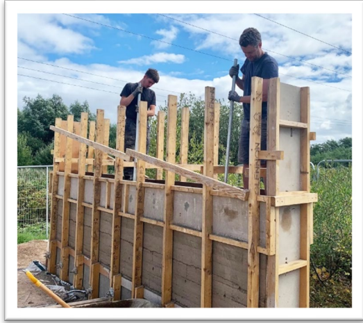
Ill. 6: Fuinneamh Workshop Architects ram an earthen wall for The KinShip EcoLab. Photo courtesy of Fuinneamh Workshop Architects, 2022.
